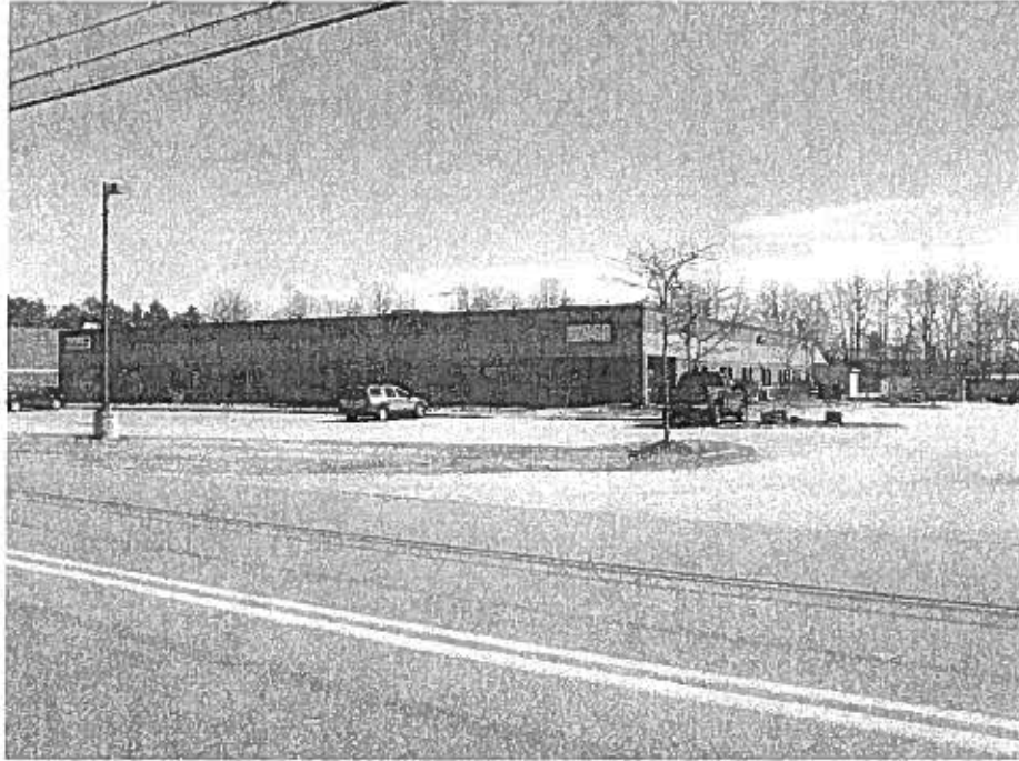
Front View from A Street - March 2010
