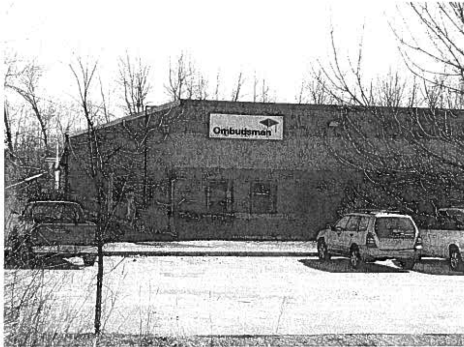
Front View from A Street - March 2010
